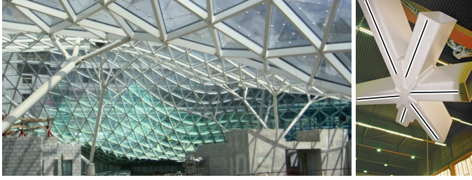
Figure 3: Complexity of nodes in triangle meshes. This image shows part of the roof of Złote Tarasy in Warsaw, designed by The Jerde Partnership, which is based on a triangle mesh, and a detail of a connector element between beams. The highlighted central lines on the beams demonstrate clearly that this is a vertex with torsion, i.e., the beams are in general position relative to each other (Photos: Waagner-Biro Stahlbau).
