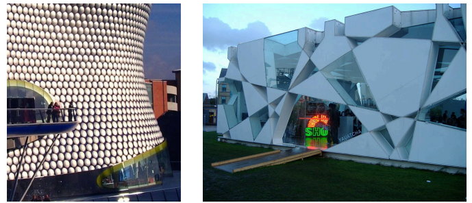
Figure 47: Patterns . Left: A pattern of circles covers Selfridges in Birmingham (2003, design by Future Systems). This pattern has regular triangular mesh connectivity, without vertices or edges being shown. Right: From the mathematical viewpoint, the 2002 temporary pavilion by Toyo Ito at the Serpentine Galleries (Hyde Park, London) has the combinatorics of a so-called arrangement of lines.
