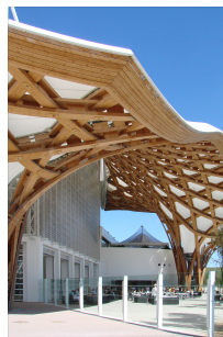
Figure 36: Wooden support structure, Centre Pompidou in Metz (France) by architect Shigeru Ban, and engineered by Arup in 2008. Production of the curved members was by CNC machining, with an estimated 50% of the raw material being chipped away during the process (photo: Annie Dalbéra).
