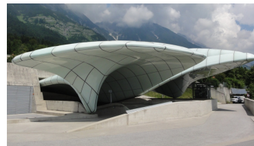
Figure 20: Double-curved glass panels with neoprene seals are covering Hungerburg station, one of a series by Zaha Hadid, built for the Innsbruck Hungerburgbahn in 2004 (photo: Wikipedia user Mattes).
