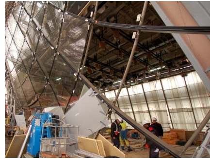
Figure 33: The Eiffel Tower Pavilions feature beams with rectangular cross-section whose side flanks are manufactured by bending. This makes them developable, and makes the entire beam arrangement a semidiscrete version of the support structure of Fig. 30, left (image: Evolute).
