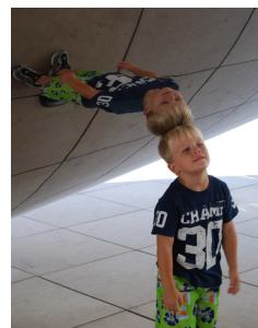
Figure 21: Reflections prove smoothness visually. The Cloud Gate sculpture by Anish Kapoor (Chicago 2006) has a seamless metal cladding (photo: Tim Schapker). Compare this image with Figure 23, where kinks in the reflection lines (at strip boundaries) reveal curvature discontinuities of the surface.
